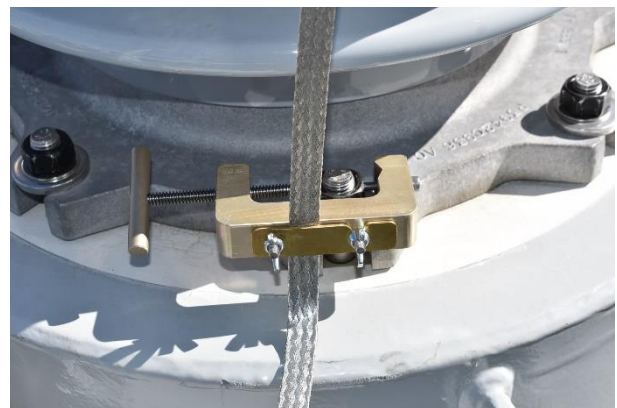
Earth connection to the ground clamp
